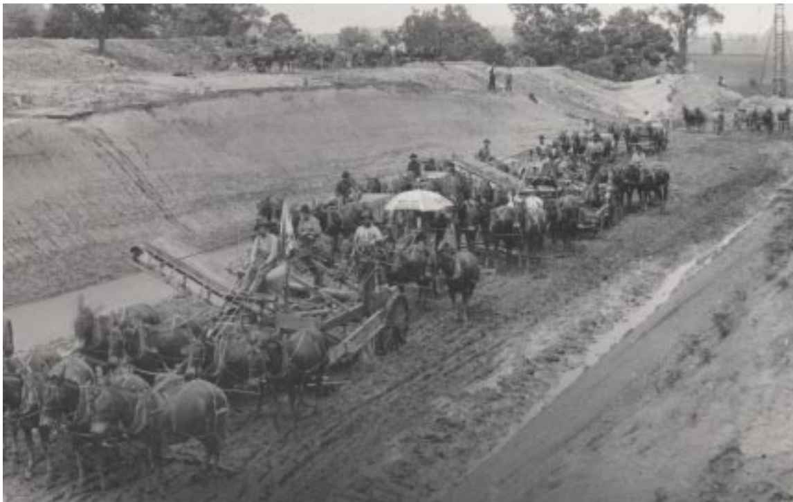
Figure 3 – Early Illinois dredging using horses
